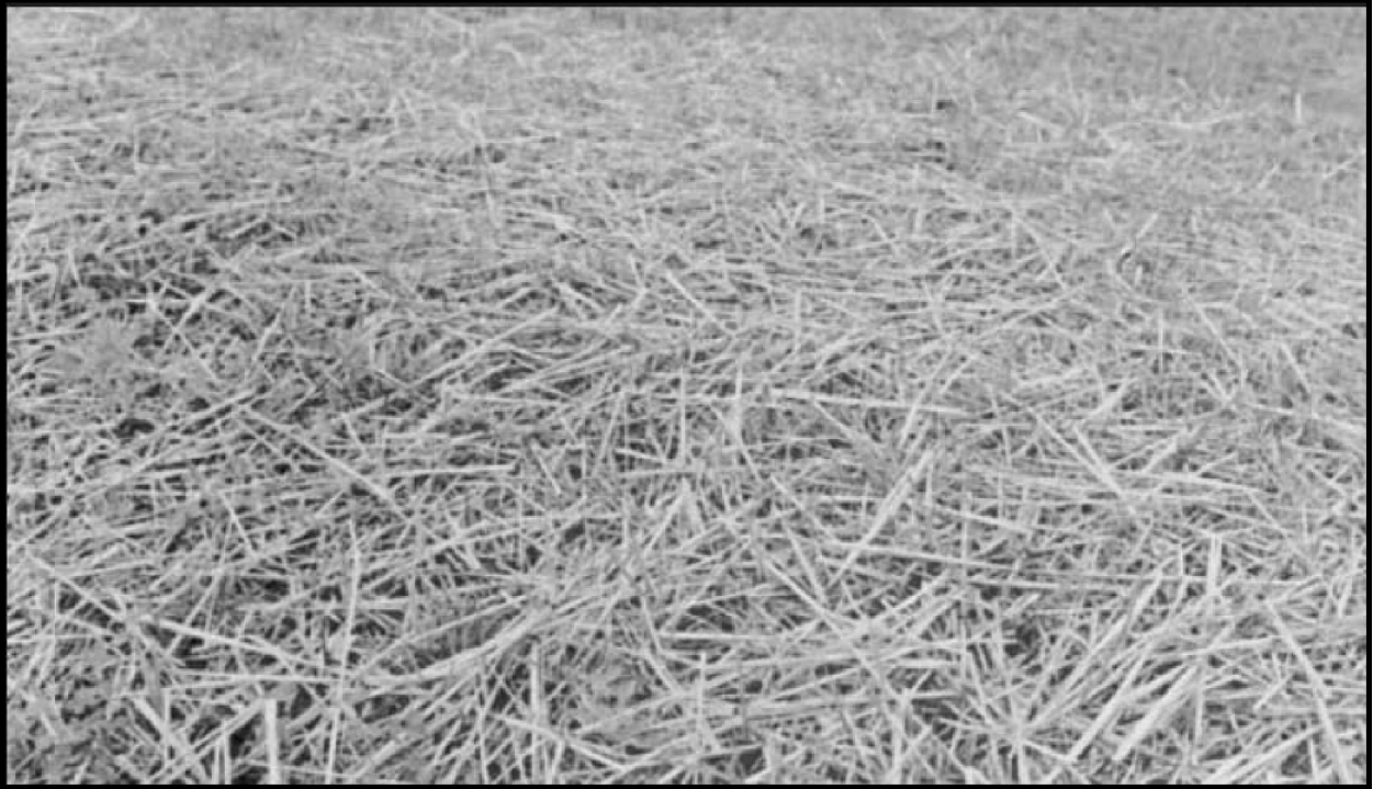
Figure 6.27 It takes about two tons per acre of straw mulch to cover at least 75 percent of the ground surface. To prevent erosion and provide the best microclimate for seed establishment, straw mulch should be physically anchored (crimped) or tied down with a tackifier.
