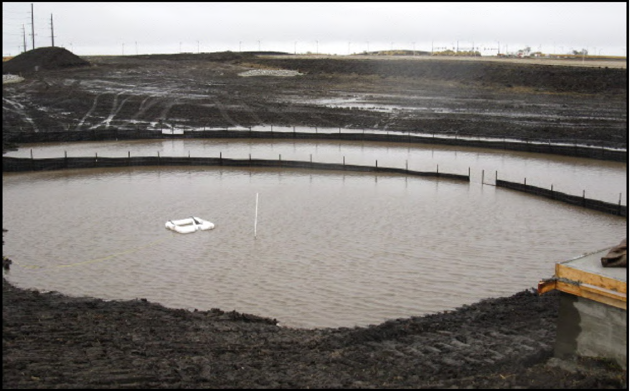
Figure 8.89 A sediment basin can be used to pretreat sediment-laden water before it discharges from the construction site. Source: BFA Inc.
