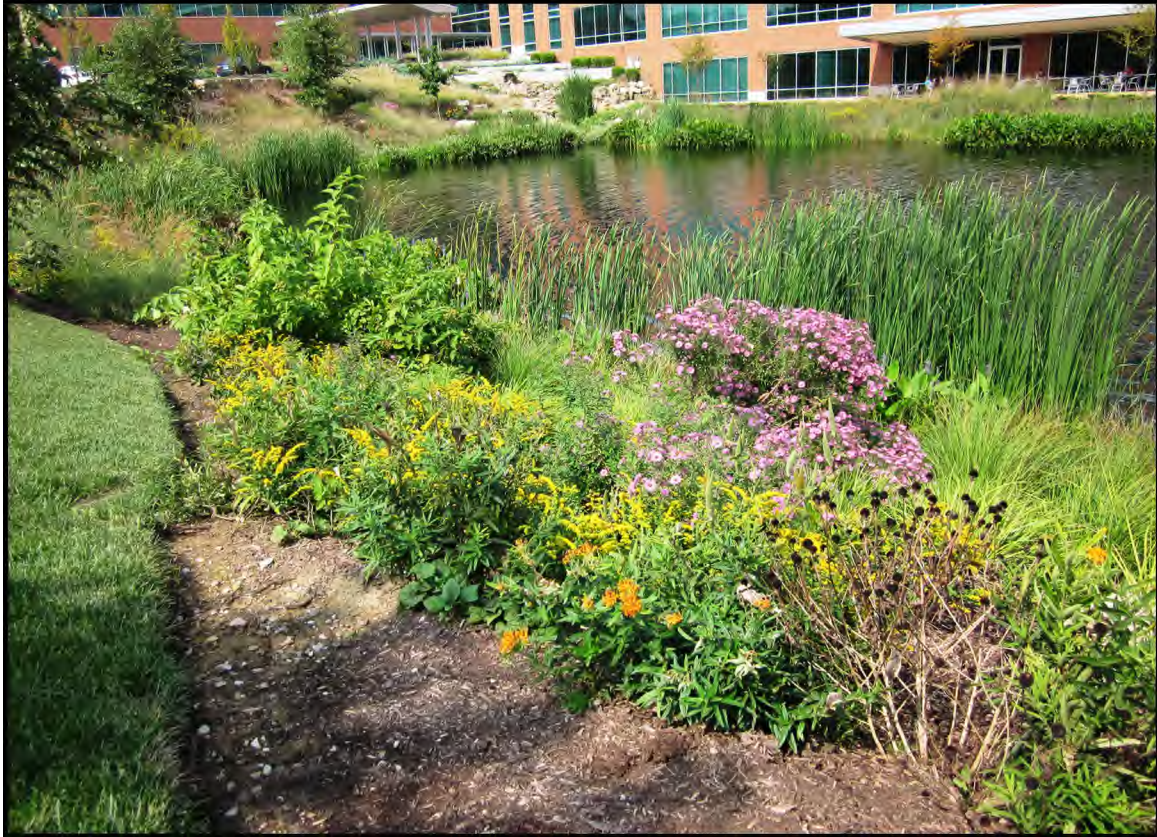
Figure 6.123: Extended Wet Detention, Express Scripts Campus, Berkeley, MO. Source: Metropolitan St. Louis Sewer District
