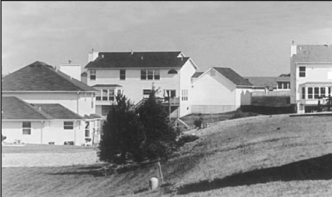
Figure 6.13 Lot benching can shorten slope length and prevent erosion while improving the homeowner's yard. Source: C. Rahm, NRCS, St. Charles County
