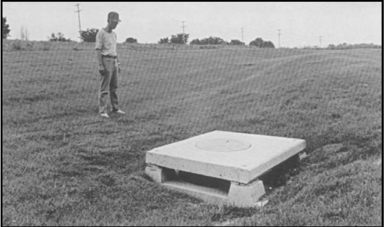
Figure 6.25 Permanent vegetation can be used to stabilize many structures, such as this grassed waterway, ensuring that runoff is relatively sediment-free.
